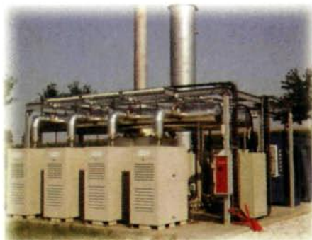
Shown is Soffimat's first landfill gas-fueled 240 kW microturbine combined heat and power array. Photo courtesy of Capstone Turbine.
